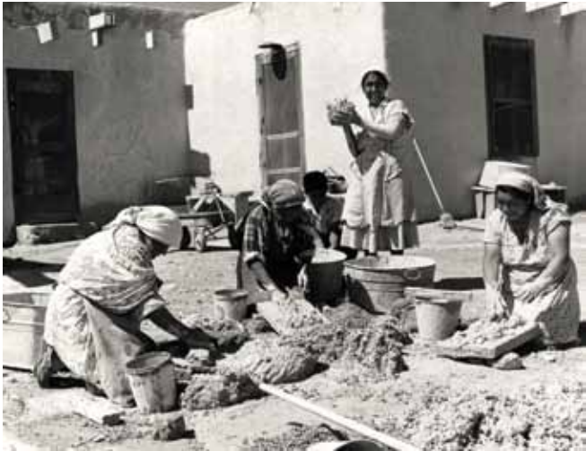
Laguna Women Plastering (1955)
